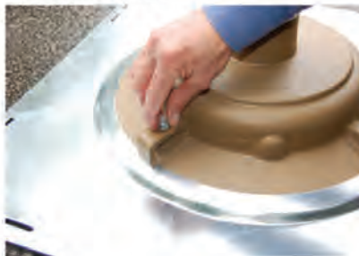
3. Bolt the 4 angled steel support brackets onto the roof drain until the deck plate is locked into place. (See -DPK Trim Kit)
