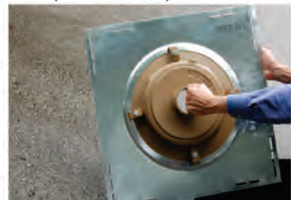
4. Place the deck plate and roof drain combination on the roof and attach the deck plate to the roof structure.
